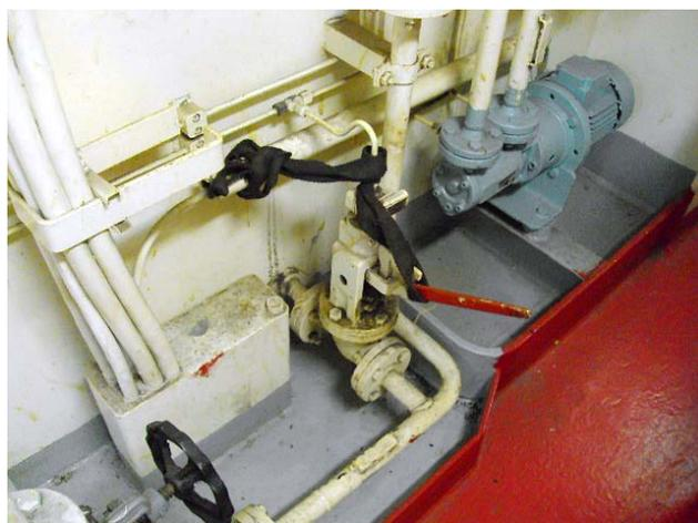
Quick Closing Valve held open with strop
