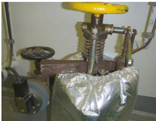
Quick Closing Valve gagged with steel wedge
